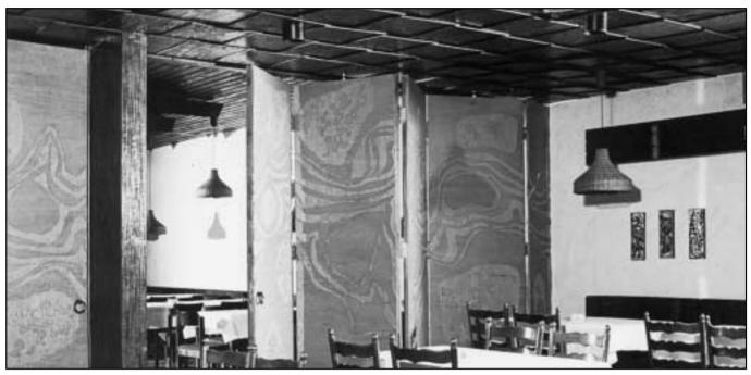
Fig. 1 Centre-folding, i. e. half inward and half outward.
